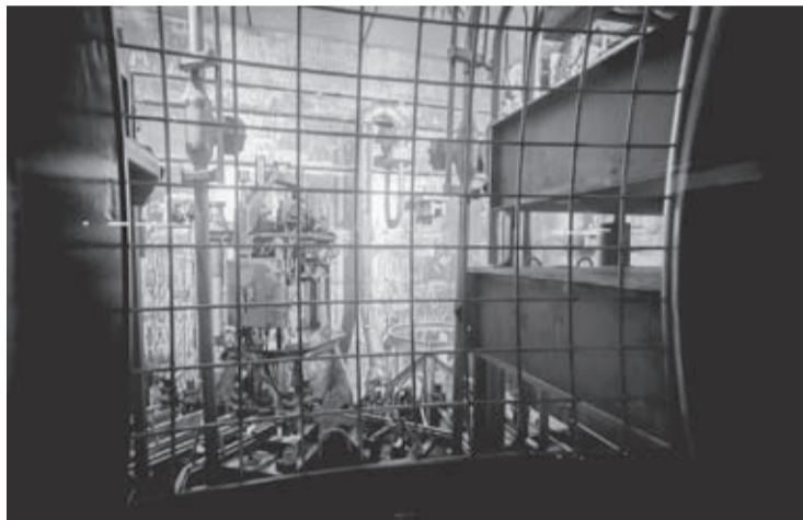
In this Nov. 20, 2013 photo, seen through thick protective glass, shows the area where workers sand-blast the large stainless steel tanks used in the vitrification process to rid them of contaminants at the Defense Waste Processing Facility at the Savannah River Site near Aiken, S.C.
